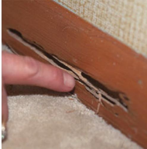
Termite damage to baseboard. Hidden infestation was discovered when vacuum cleaner attachment penetrated surface of baseboard.
